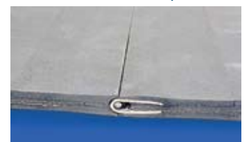
Covered splice top & bottom
